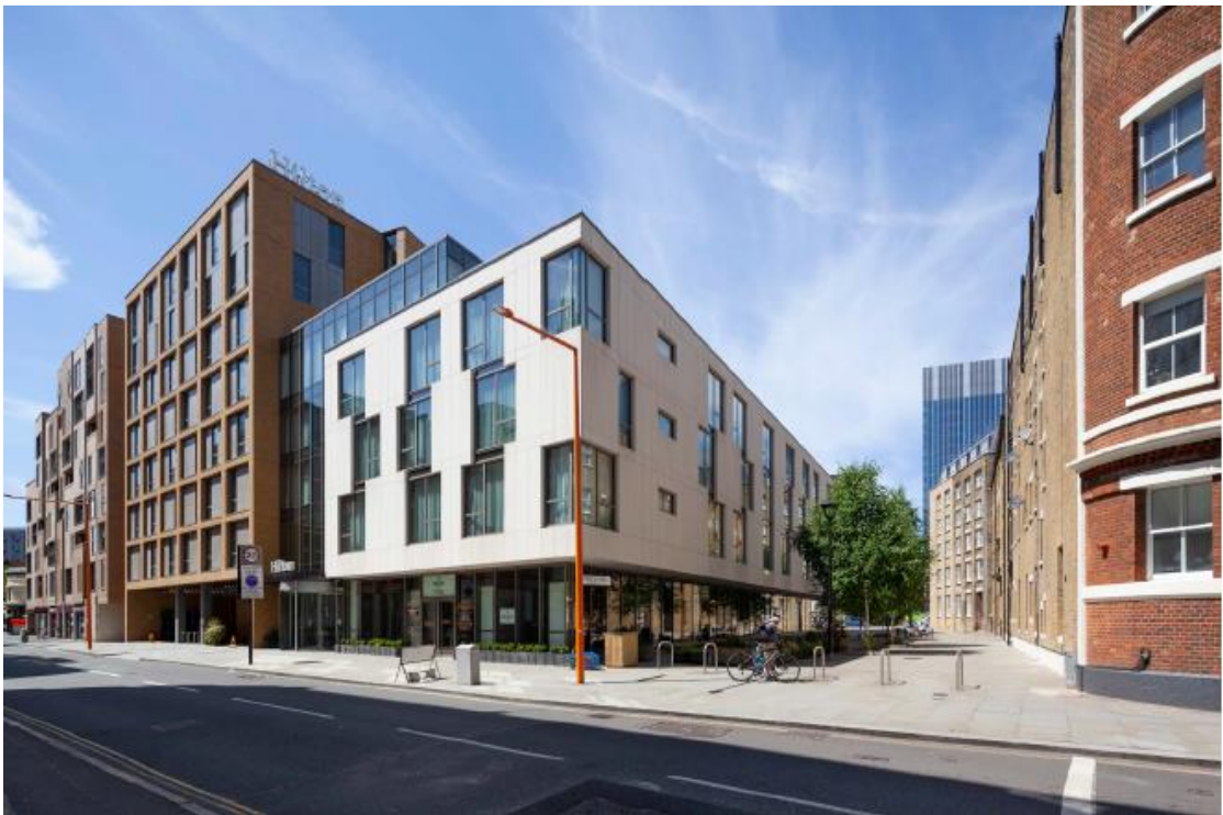
Image 2: Existing building photo view from Great Suffolk Street.
